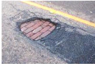
into the pavement and expands as it freezes, it pushes up on the pavement. The weight of cars and trucks then can break up this newly uneven pavement, starting a pothole.
